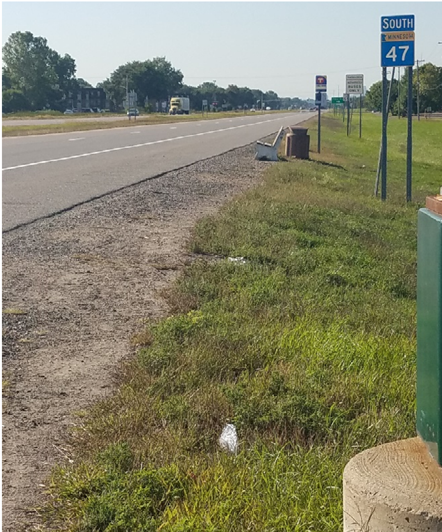
Figure 2-6: Bus Stop without Shelter at TH 47 and 81 st Avenue NE
