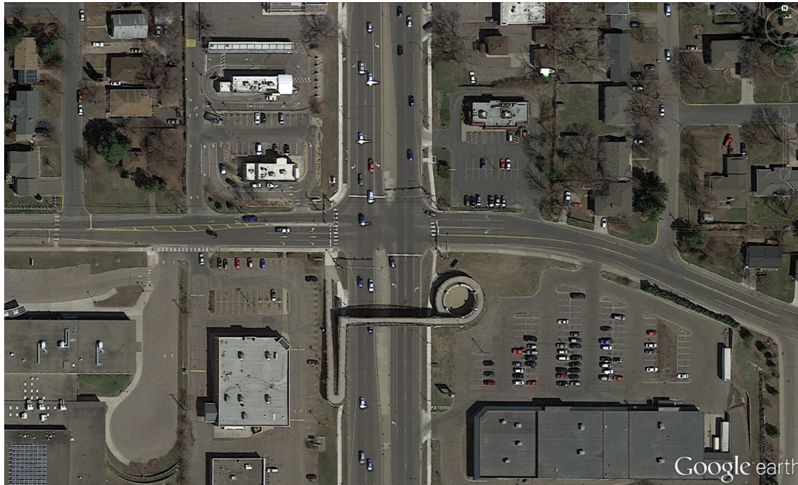
Figure 4-43: Aerial Image of 49th Avenue NE and TH 65
