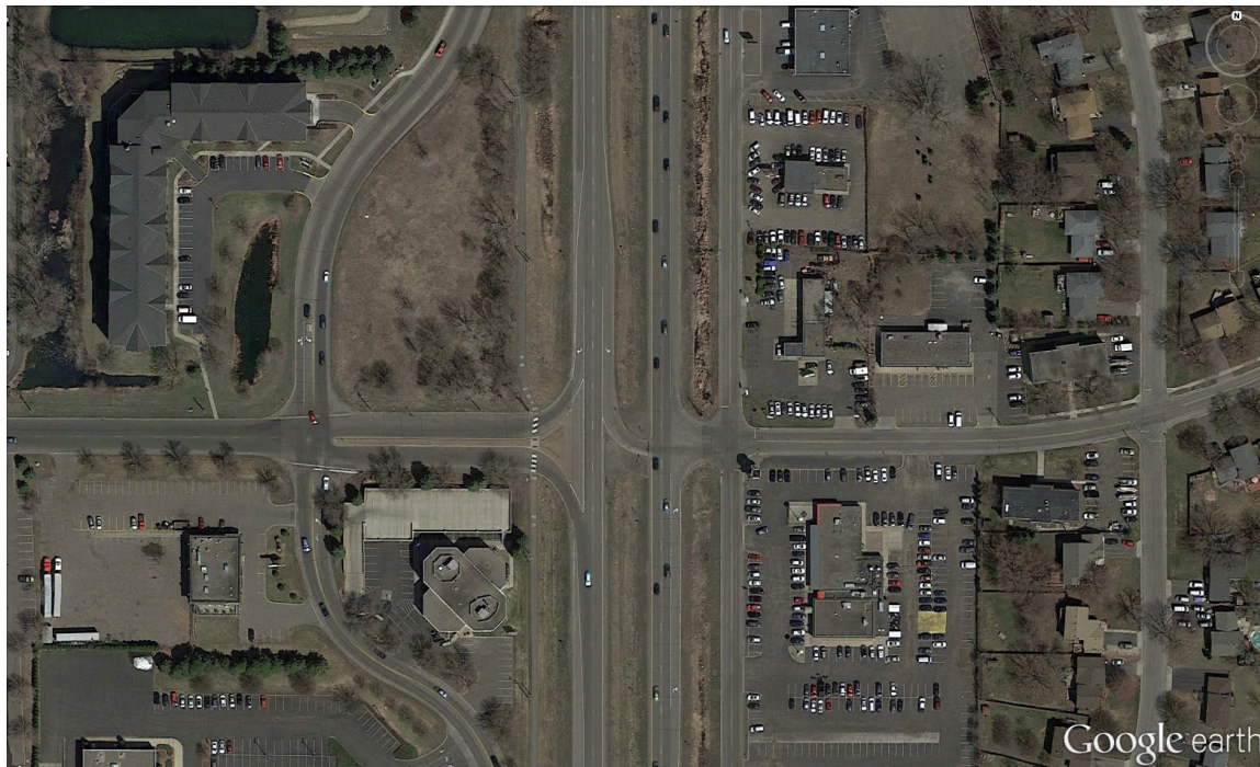
Figure 4-31: Aerial Image of 83rd Avenue NE and TH 47
