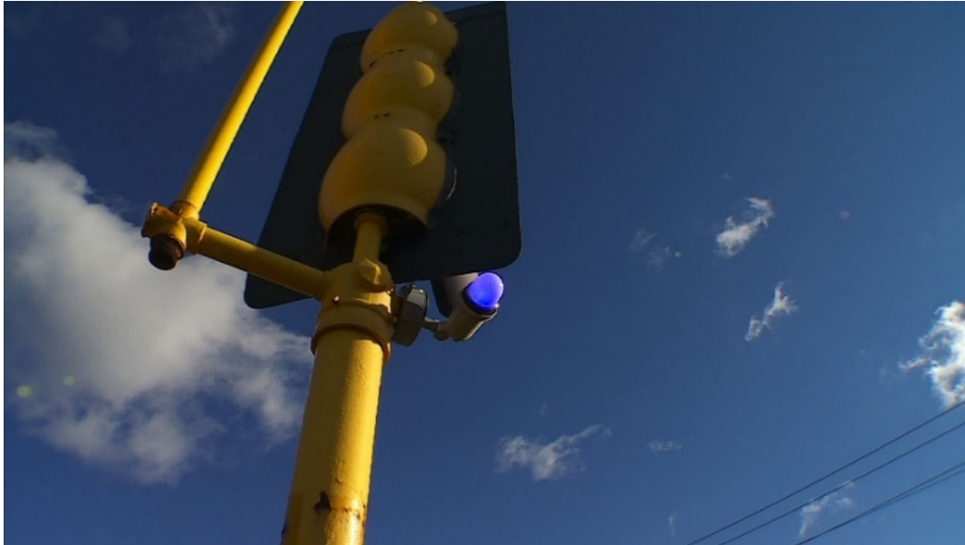
Figure 4-1: Example of Blue Light Enforcement Installed on Traffic Light
