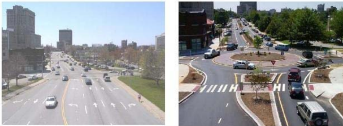
Figure 4-18: Asheville, NC, Safe Infrastructure Project (Before and After)
