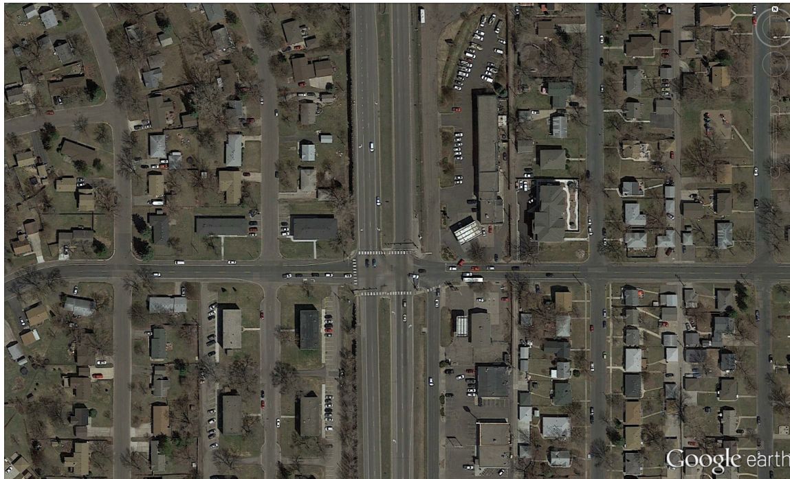
Figure 4-23: Aerial Image of 53 rd Avenue NE and TH 47
