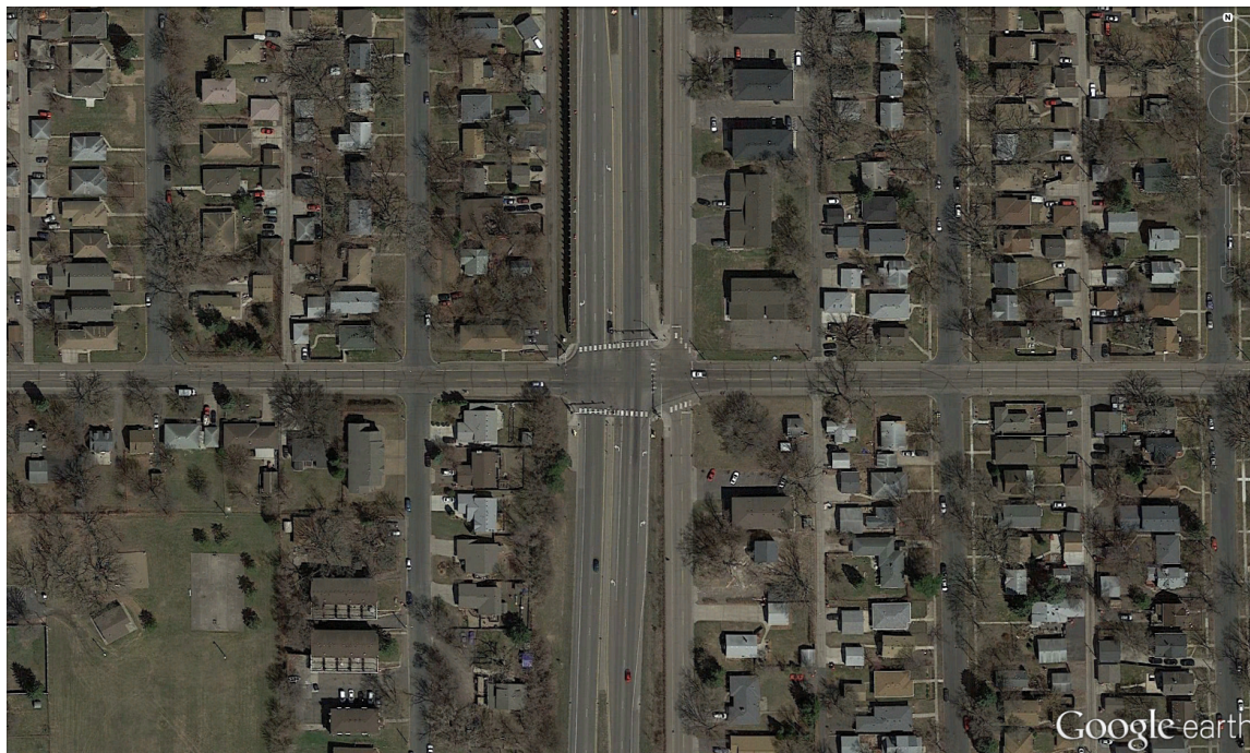
Figure 4-21: Aerial Image of 44th Avenue NE and TH 47
