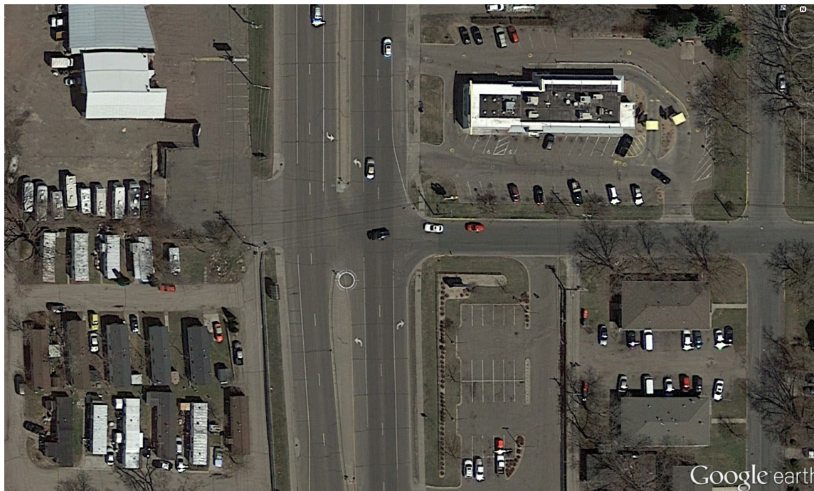
Figure 4-41: Aerial Image of 46th Avenue NE and TH 65
