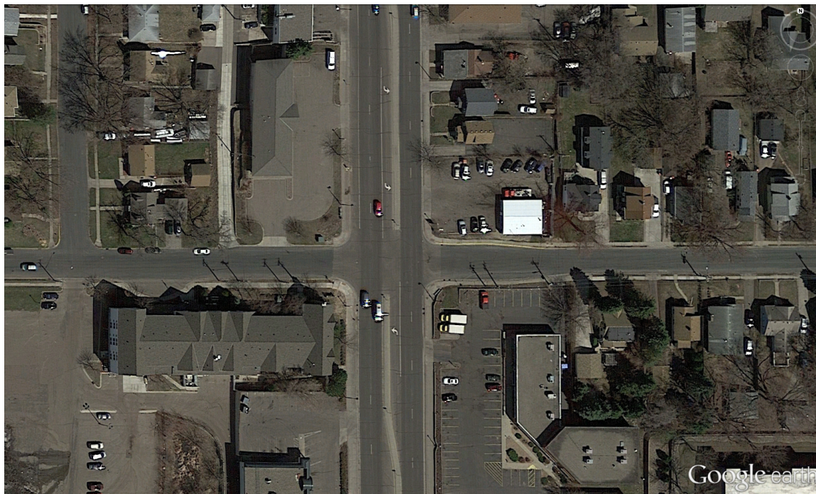
Figure 4-37: Aerial Image of 42nd Avenue NE and TH 65
