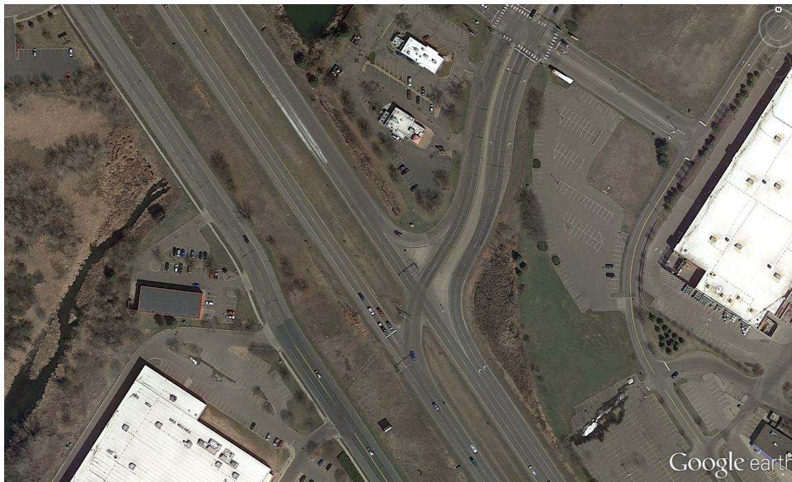
Figure 4-33: Aerial Image of University Avenue NE and TH 47
