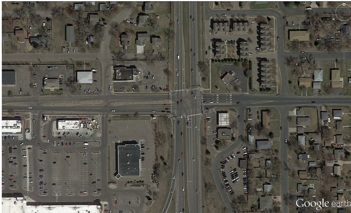
Figure 4-26: Aerial Image of 57th Avenue NE and TH 47
