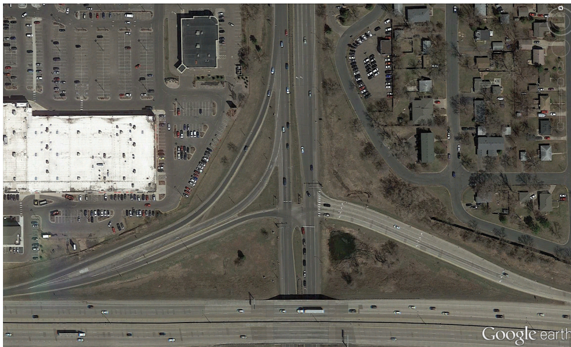
Figure 4-25: Aerial Image of I-694 North Ramp Terminal and TH 47
