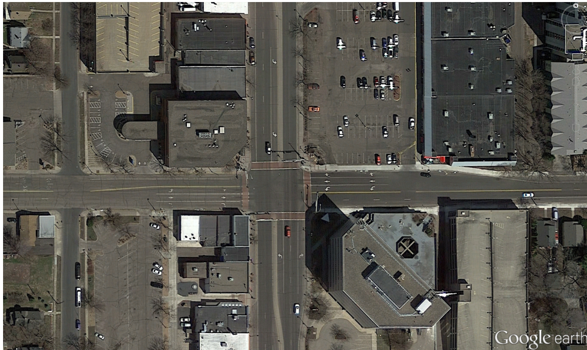
Figure 4-36: Aerial Image of 40th Avenue NE and TH 65
