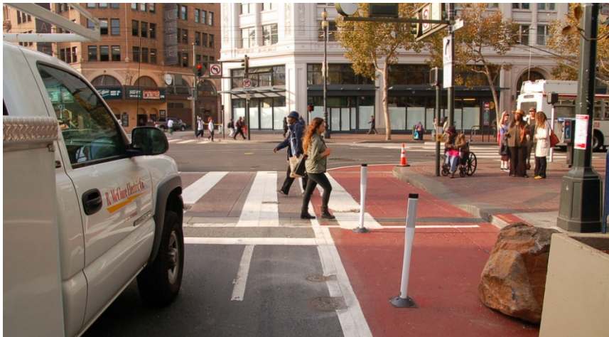
Figure 4-7: Temporary Bump Outs
