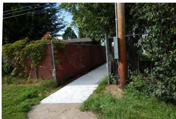
View of pedestrian pathway at the north side of school grounds (see location D on the following page).
