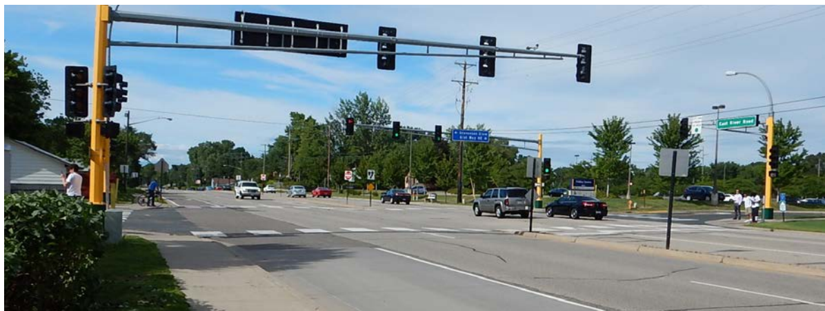
View of East River Road looking north past 61st Way NE. Pedestrians must cross seven lanes of traffic to reach the opposite side of the street. No median refuge large enough to safely and comfortably accommodate pedestrians.
