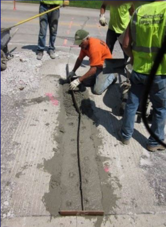
Type B3 Crack Repair
