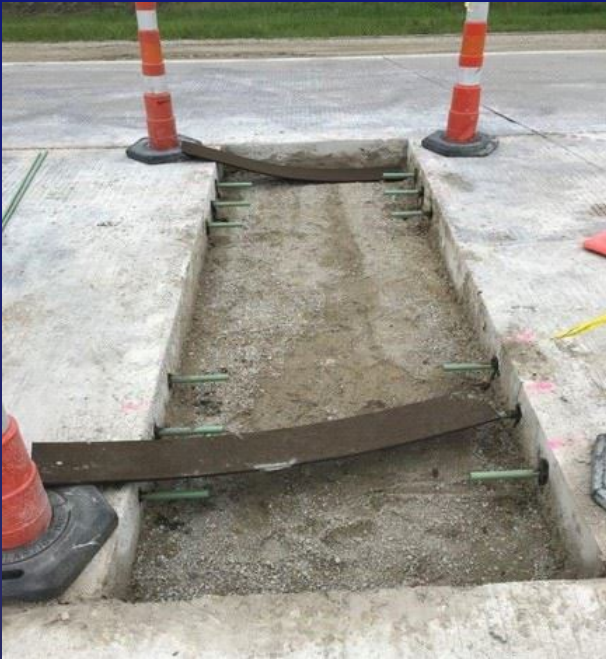
Type CD-LV Full-Depth Repair
