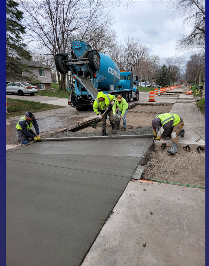
Concrete Pavement Rehabilitation
