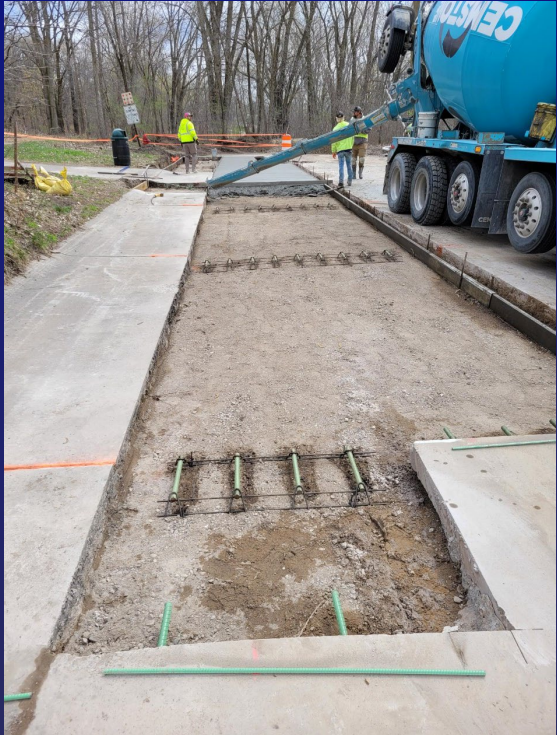
Type CX Full-Depth Repair
