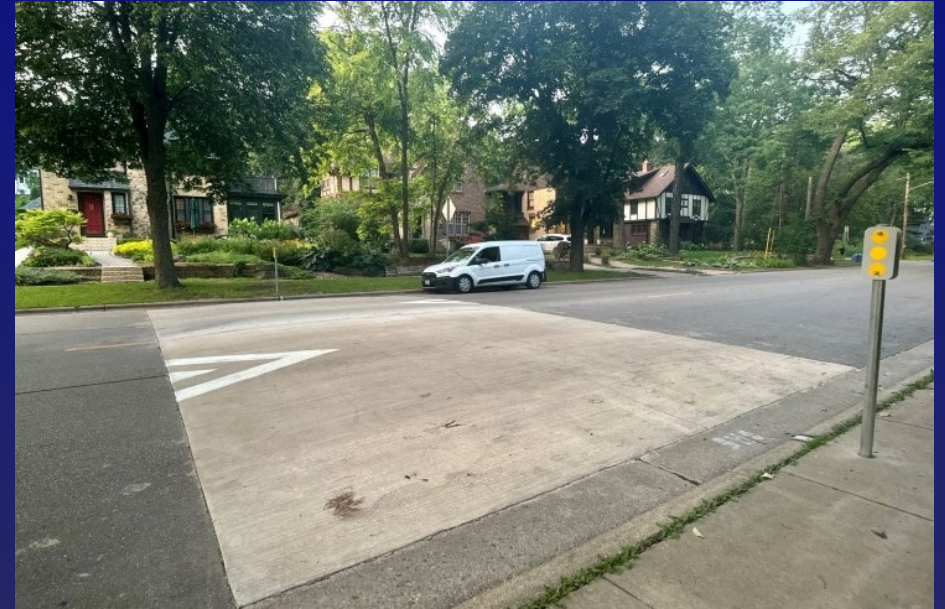
Concrete Speed Hump
