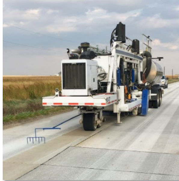
Concrete Surface Grinding
