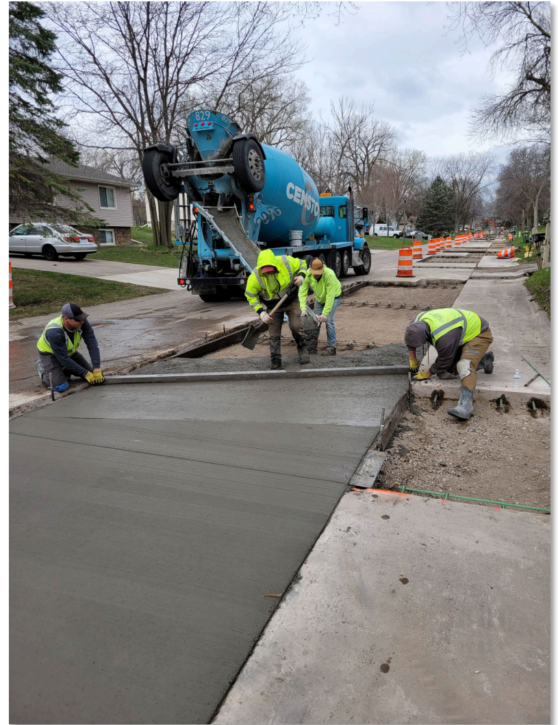
Full-Depth Concrete Pavement Rehabilitation
