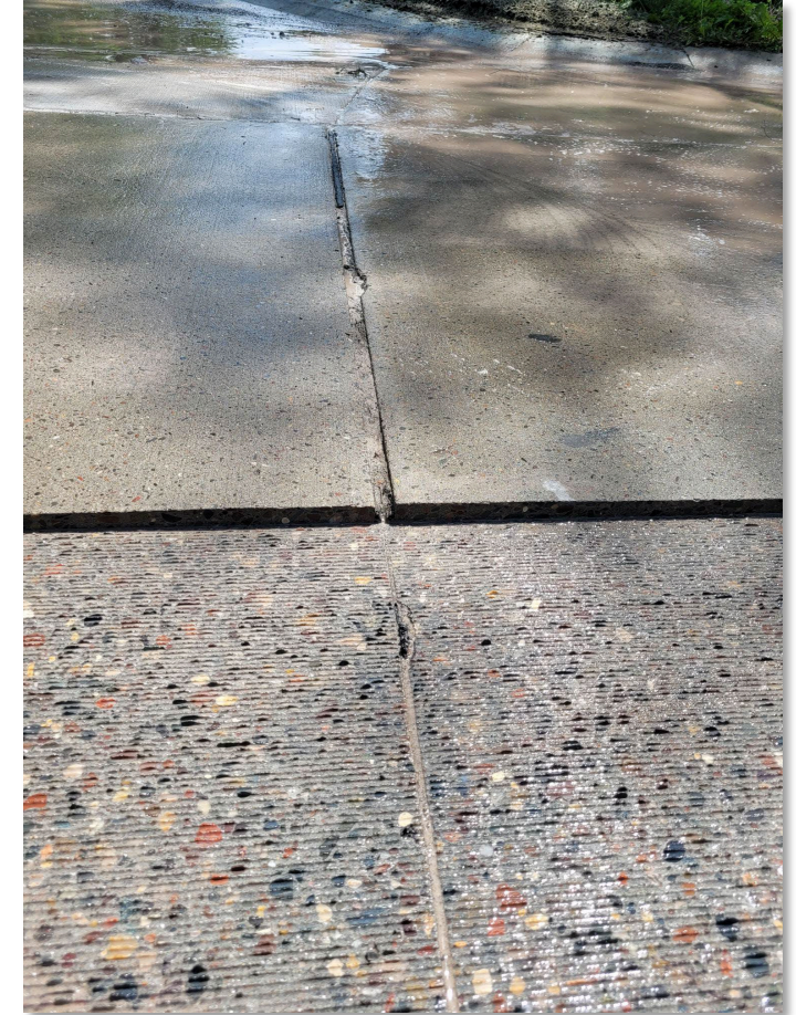
Before vs. After Concrete Surface Grinding
