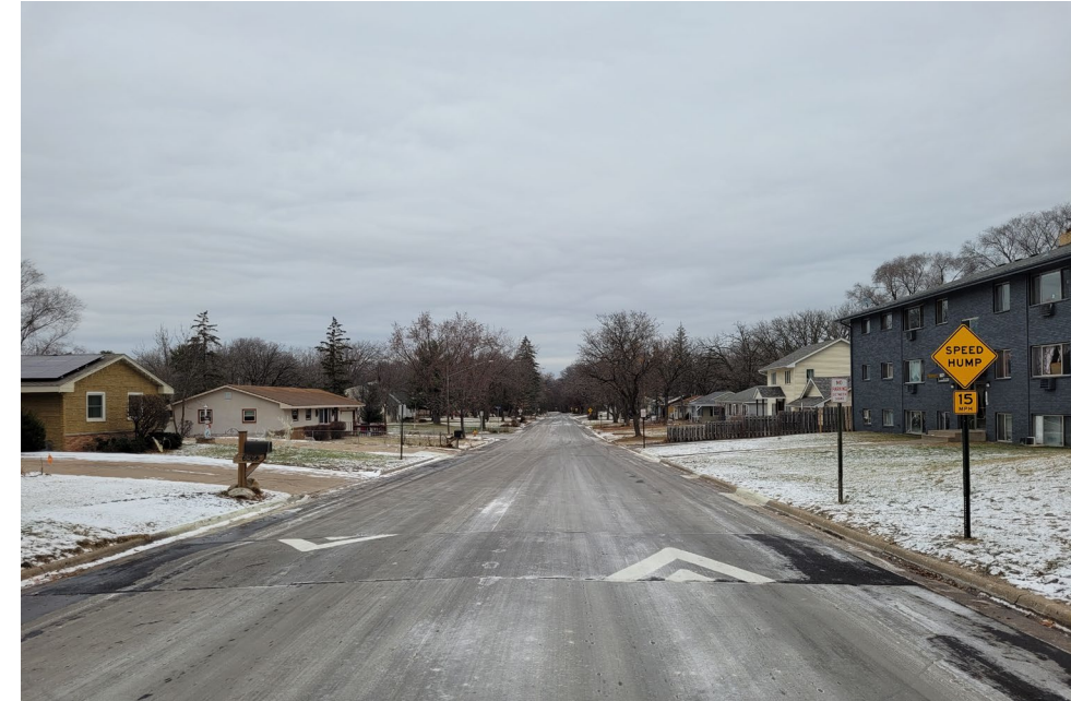
Speed Hump (Channel Road, Fridley)
