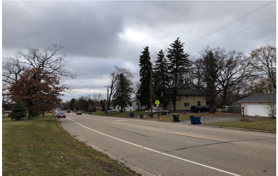
Gardena Avenue Crossing
