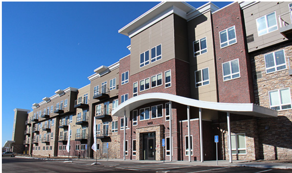
The Cielo Apartments Phase I - April 2016
