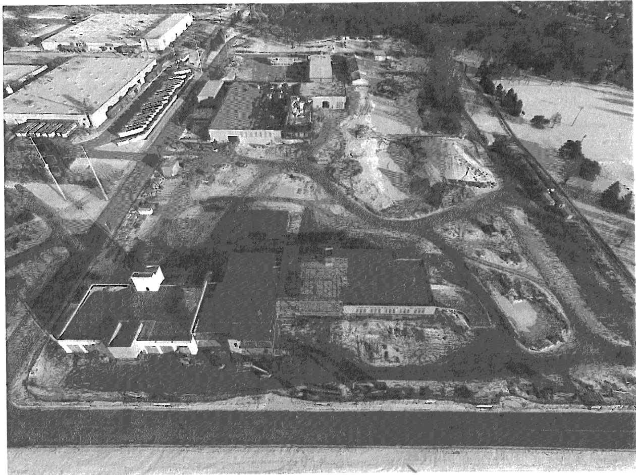
Civic Campus under construction, December 2017
