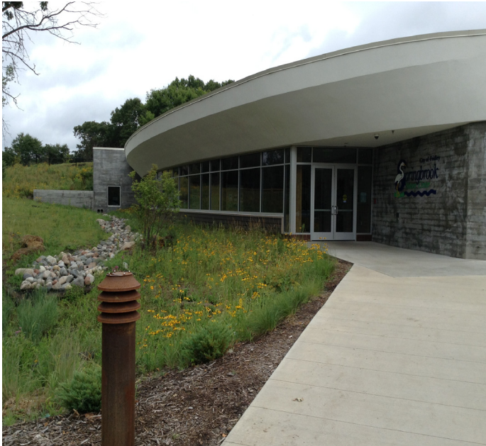
Springbrook Interpretive Center, Native Landscaping
