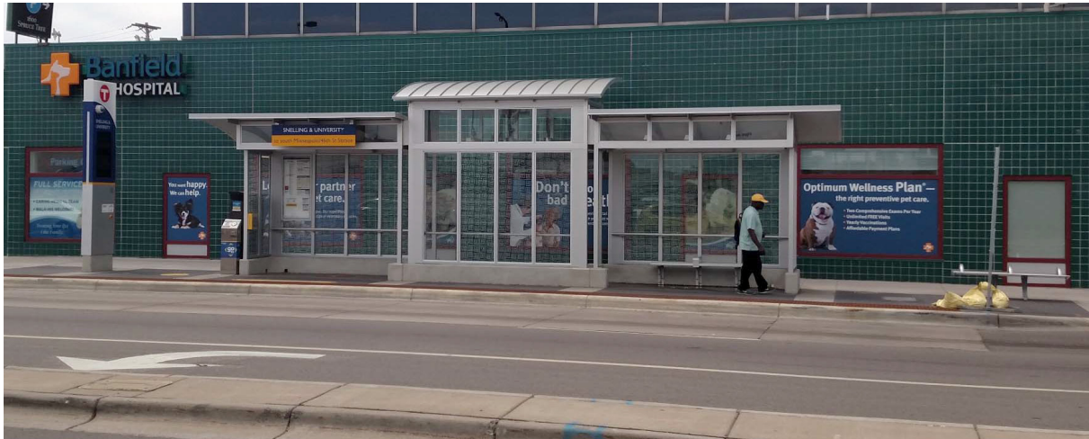
Existing BRT Stop Snelling and University in St. Paul, Photo provided by Metropolitan Council
