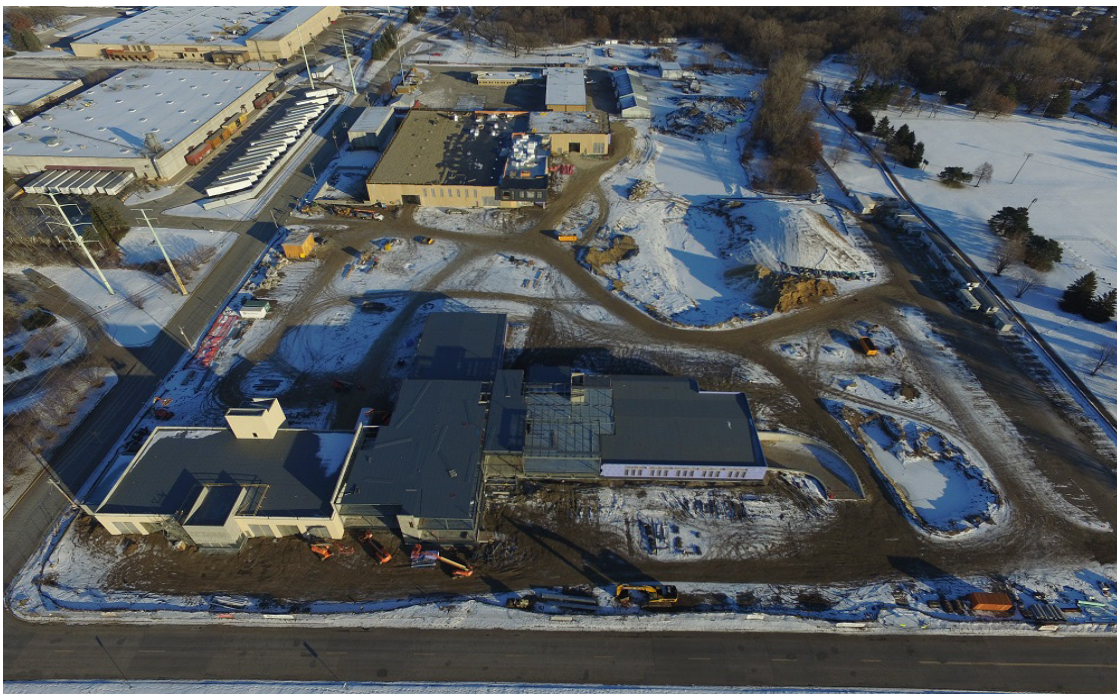
Civic Campus Construction, December 2017, photo by Ryan Wickstrom
